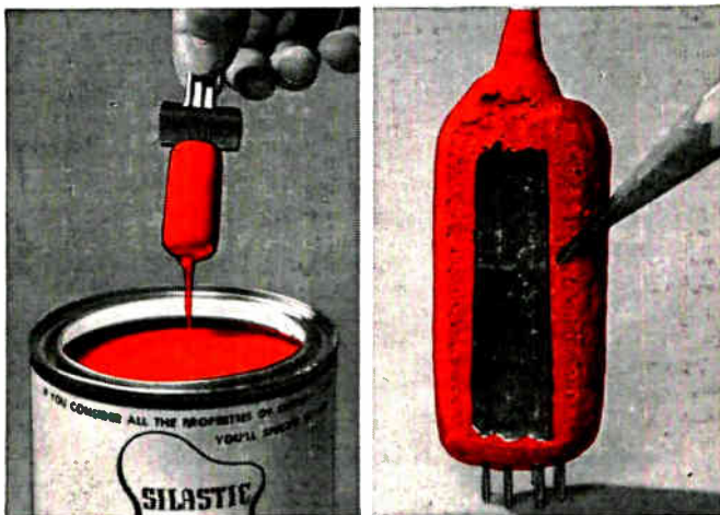
Electronic tube encapsulated with Silastic.
