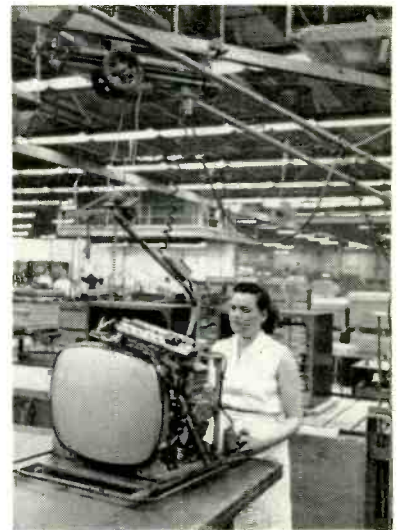
Cylinder shoulders weight of chassis
