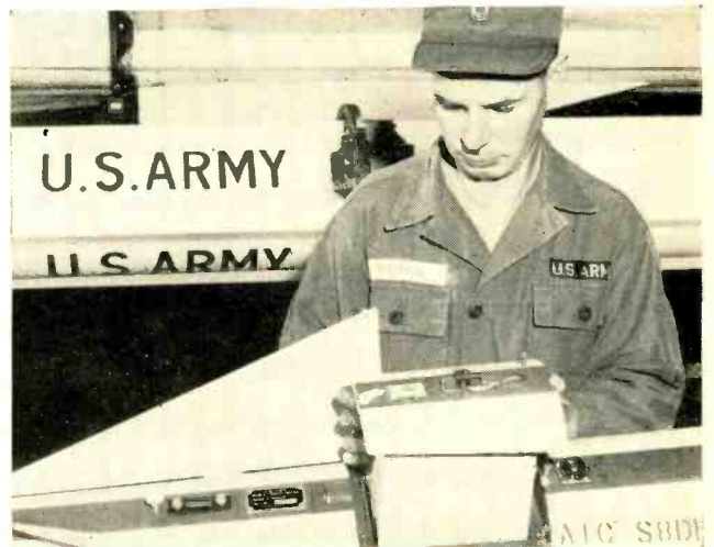
Army technician checks battery as part of routine maintenance on Nike missile installation. Reliability is strong factor in the design of modern batteries for use in missiles like these. At right, battery is removed from specially designed recess for replacement
