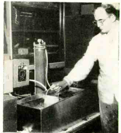
Resin water purifying unit is shown in place at a cascade washing station for electron tube parts
