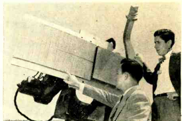
Setting the stage for new product developments, the Hughes Research & Development Laboratories delve into basic theory. Here R & D engineers work with a slot-array microwave antenna.
