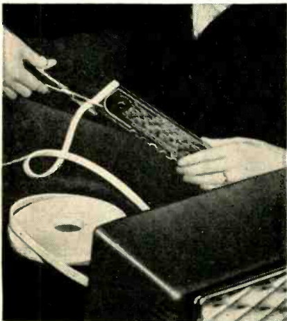
Tape is pressed on radio dial and cut with scissors, for cushioning and dust exclusion
