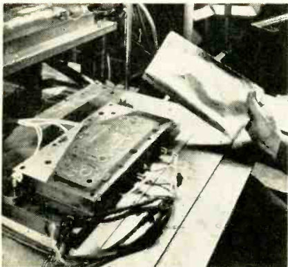
Raised pattern on heated die corresponds to desired printed wiring pattern
