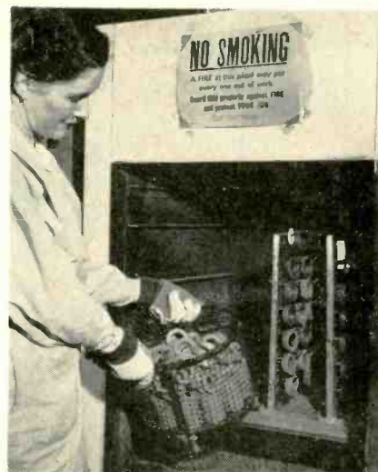
New method of drying impregnated cores in basket. Loaded rack in oven illustrates method formerly used
