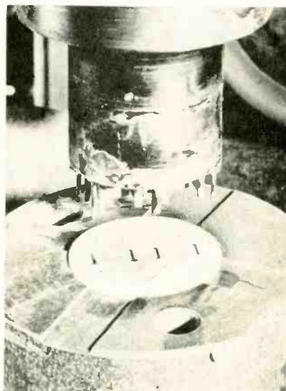
Withdrawing tool after cutting holes
