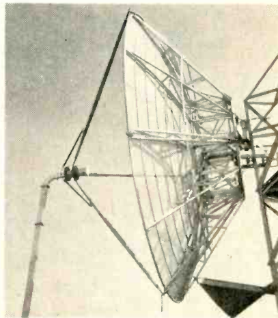
Scatter transmission system between Cedar Grove, N. J. and Somers, Conn. uses 18-ft parabolic reflector. The Du Mont system operates at 2,180 mc carrying 72 voice channels. Transmitter output is 1-kw. Receiver is dual diversity type operating reliably on an 8 microvolt signal
