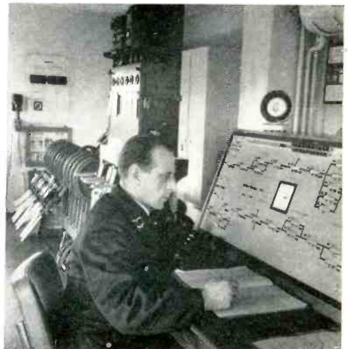
train actuate lamps at central control board (right) that shows track occupancy and progress of trains
