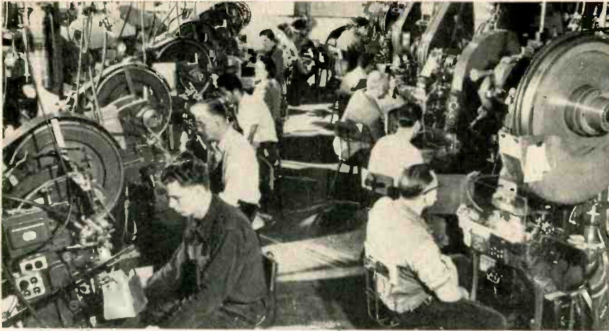
POWER presses at Volkert Stampings produce metal parts for tubes as . . .
