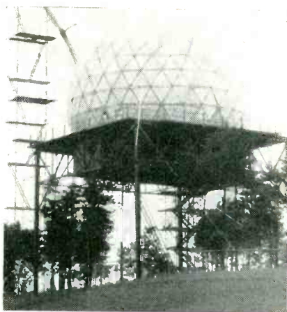
TRANSLUCENT plastic radome for DEW-line (left) and over-the-horizon antenna for White Alice (right) are latest additions as . . .
