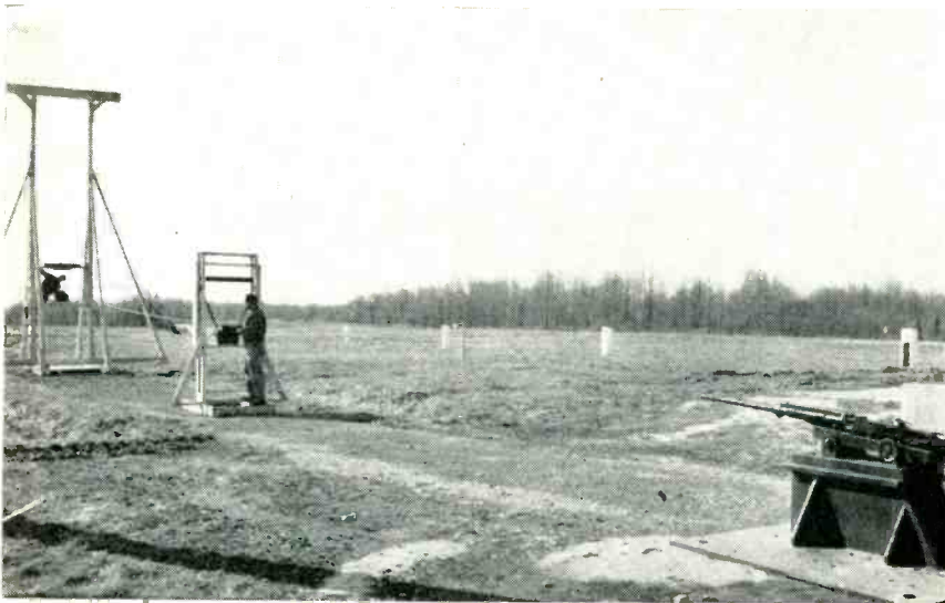
Operators measure distance between photoelectric detector screens on weapons range at Aberdeen Proving Grounds before checking projectile flight times electronically
