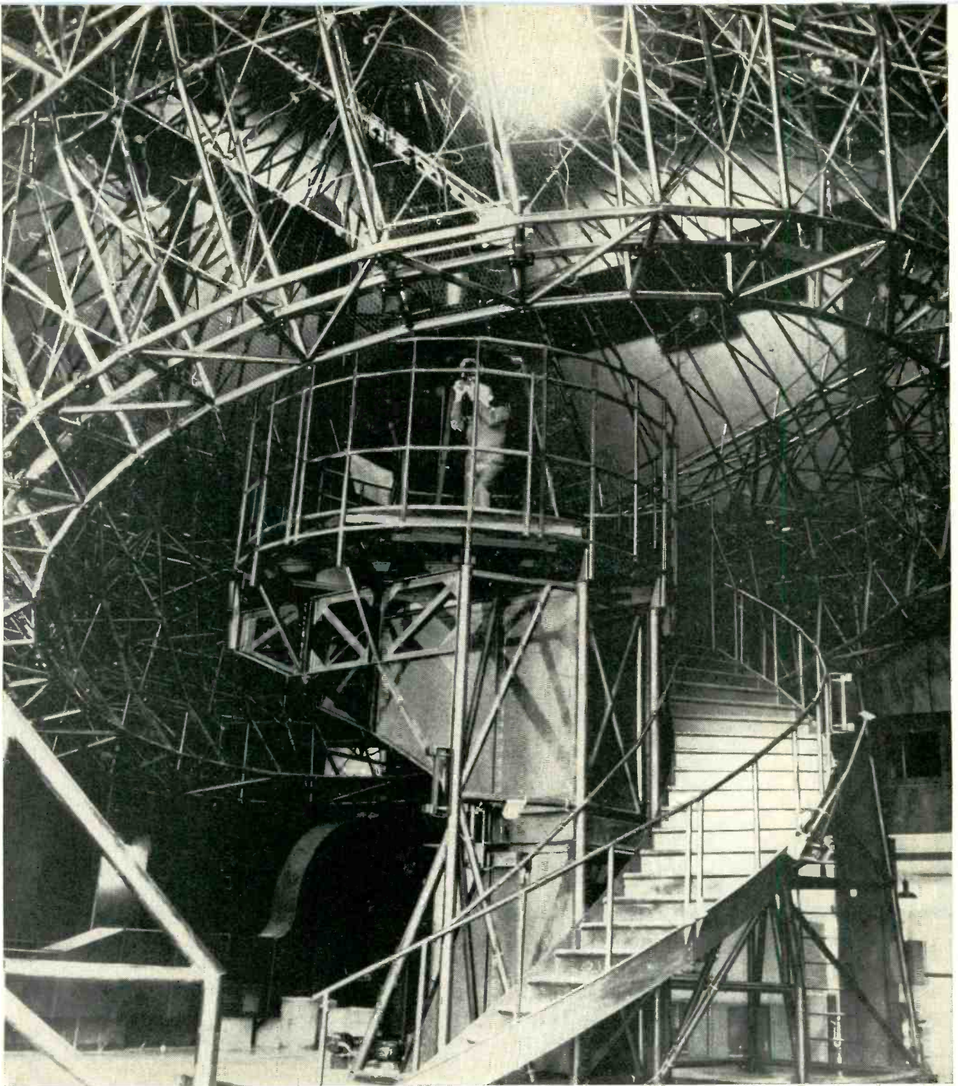
CELESTIAL NAVIGATION —Link Aviation's high-speed, high altitude celestial navigation trainer; only such trainer capable of simulating trans-Polar flight. Trains navigators in techniques of guiding planes by the stars.
