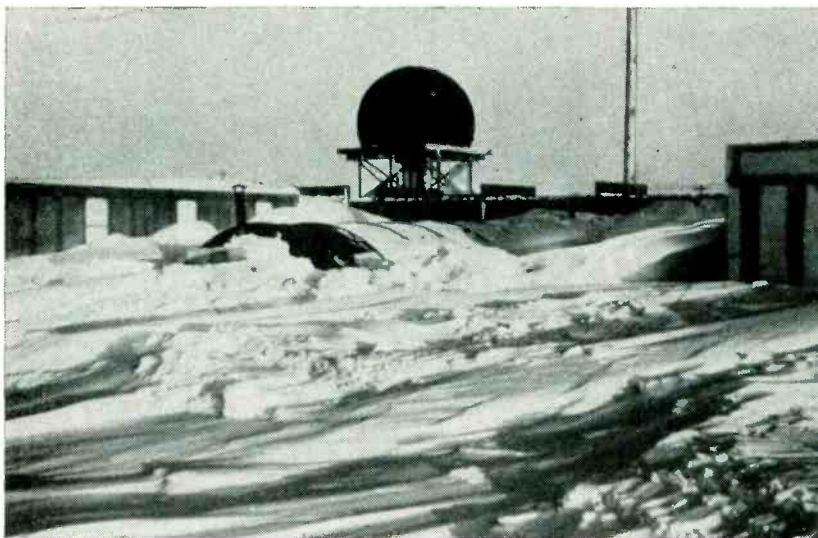
Experimental radar unit in the Arctic is prototype of those for Distant Early Warning (DEW) Line to be constructed for detection of approaching unauthorized aircraft. Mushroom-shaped rubber dome houses a radar antenna and protects it from weather. Western Electric is prime contractor
