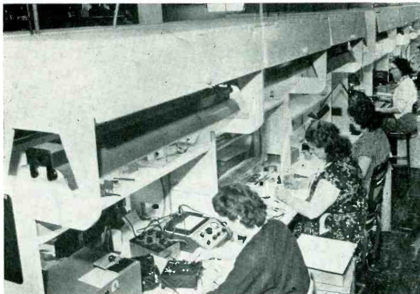
Seven-bench assembly line using unitized design. Each worker has own fluorescent fixture with two 4-foot lights, storage compartment above fixture and plywood box on floor alongside chair for tote boxes. Utility connections are on ceiling
