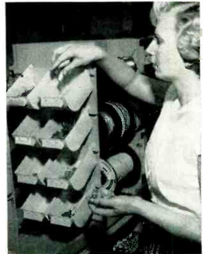
Method of swinging hinged parts rack for replenishing stock from rear
