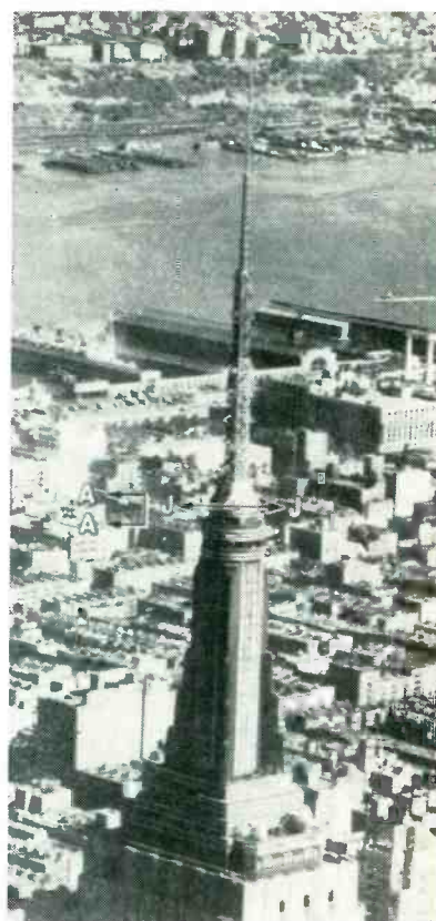
Empire State Building before construction of WOR-TV antenna showing space available for installation
