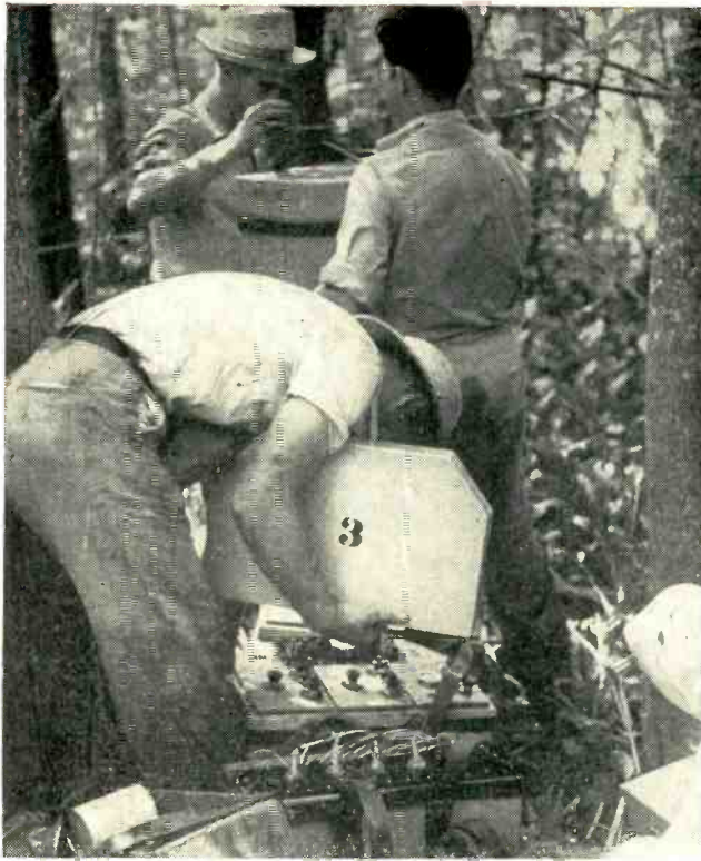
Seismic crew, left, unpacks portable amplifiers while operator, right, inserts photographic paper leader into recording oscillograph that is fed by the geophone amplifiers
