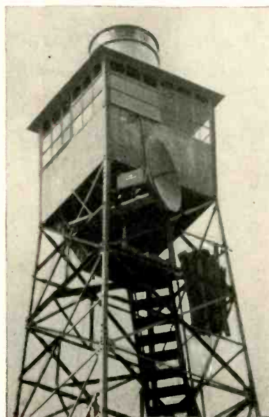
Rotating camera on top of unattended fire tower scans surrounding area and sends image through Raytheon microwave link to central observing stations
