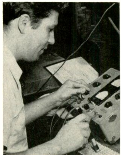
Setup for checking diodes that are still in their corrugated shipping tray
