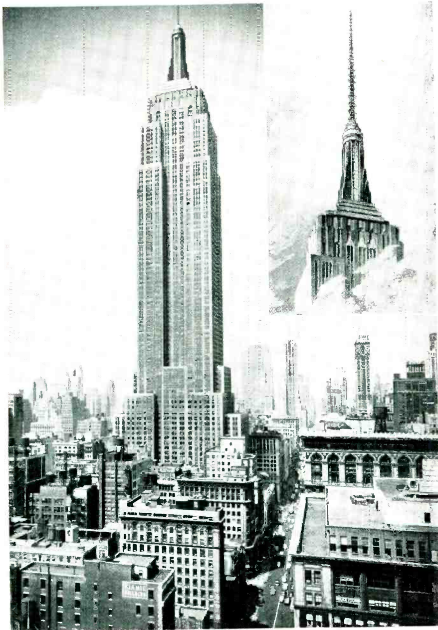
New York's 1,250 foot Empire State Building as it looked when topped by WNBT's 32-foot pole and, in the insert, architect's sketch of the new 222-foot structure which will serve five television stations
