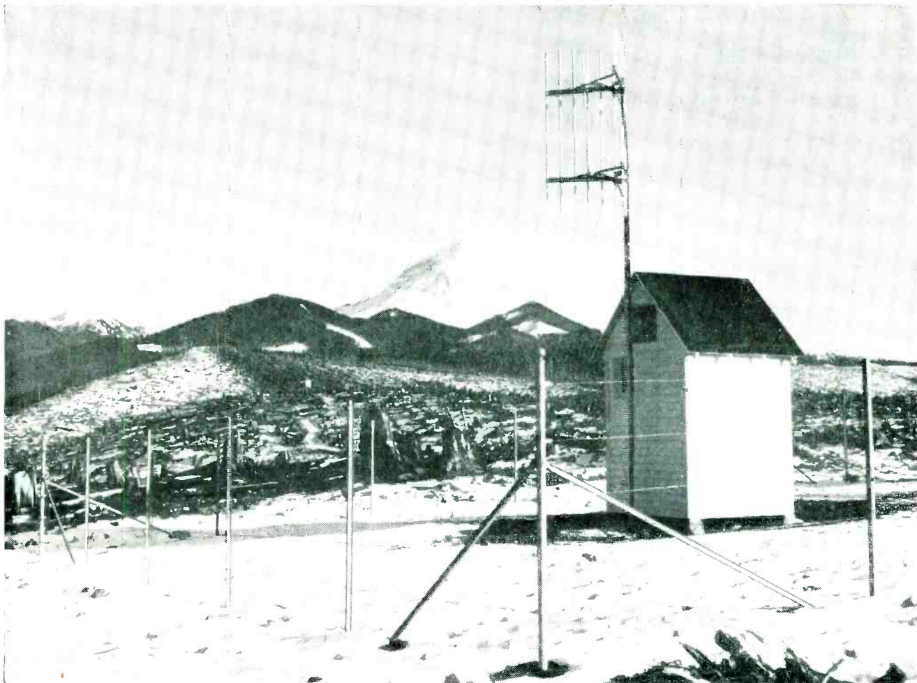
Typical unattended repeater that receives signals from several radioactive-snow-gage data-transmitting stations located in remote mountain areas and relays them to a more accessible recording station
