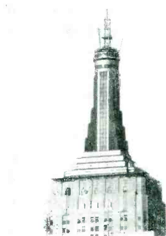
The first mast section was assembled piece by piece as it rose with the aid of the movable scaffold and a small but sturdy crane
