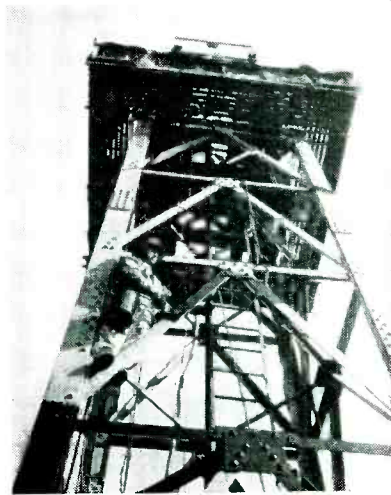
A scaffold encircling the mast went along as 57 tons of steel capable of withstanding at least 110 mph of wind pressure moved skyward
