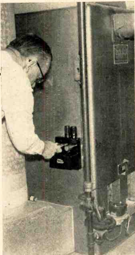
Replacing tube in electronic control unit for gas furnace in home
