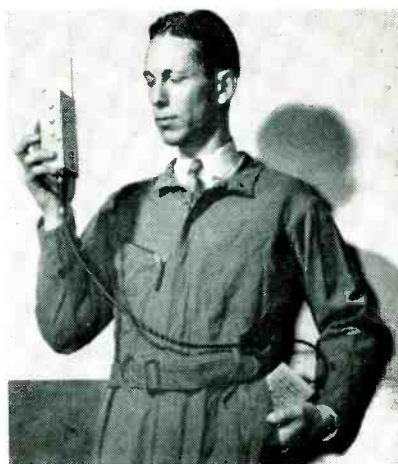
J. S. Horrigan, USAF's Air Materiel Command project engineer on the URC-4, demonstrates how the battery of the midget air-sea rescue transmitter-receiver can be slipped into the pocket of an ordinary flying suit
