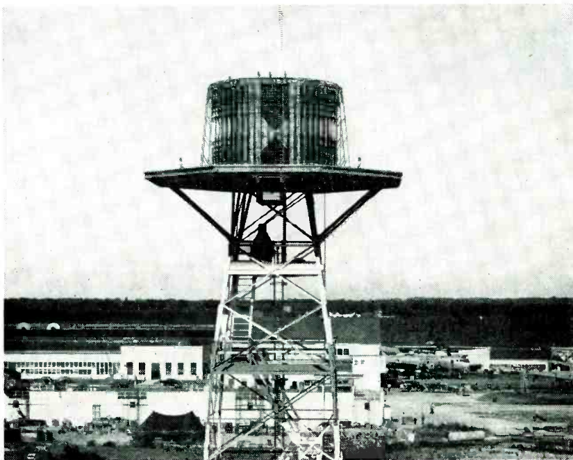
Circular lens antenna for shf consists of metal slats that direct 6-cm waves toward horizon, avoiding ground reflections. Supporting tower is 75 feet high
