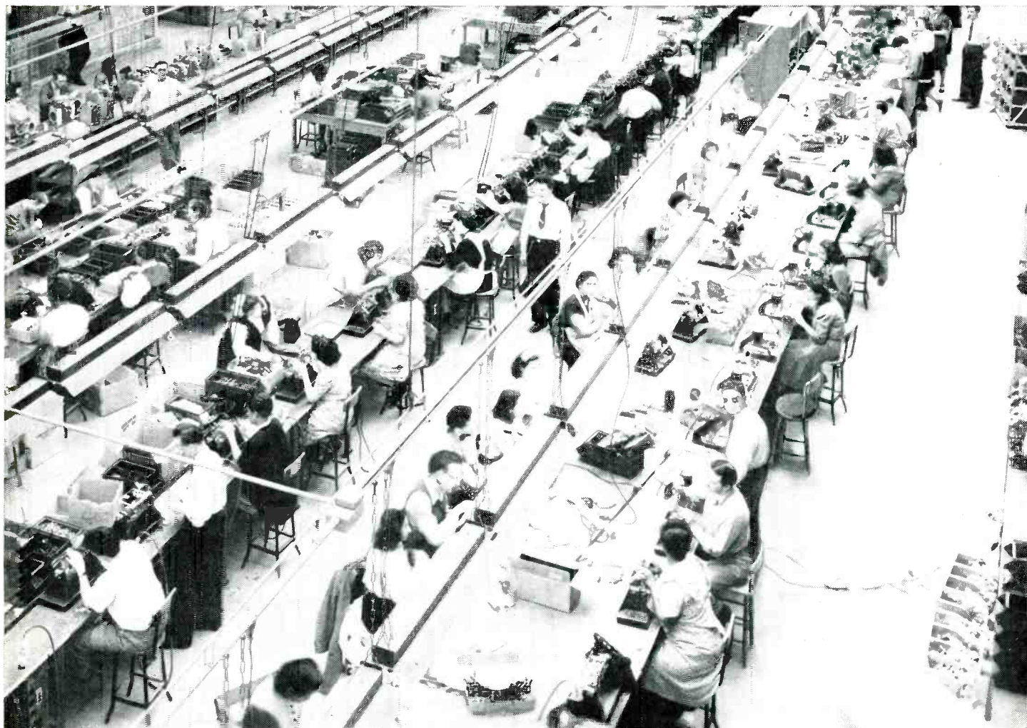
Production lines in a typical receiver assembly plant, illustrating use of over-head trolley-duct wiring, rail-guided chassis cradle, soldering-iron fixture and other cost-reducing methods and fixtures described in this article
