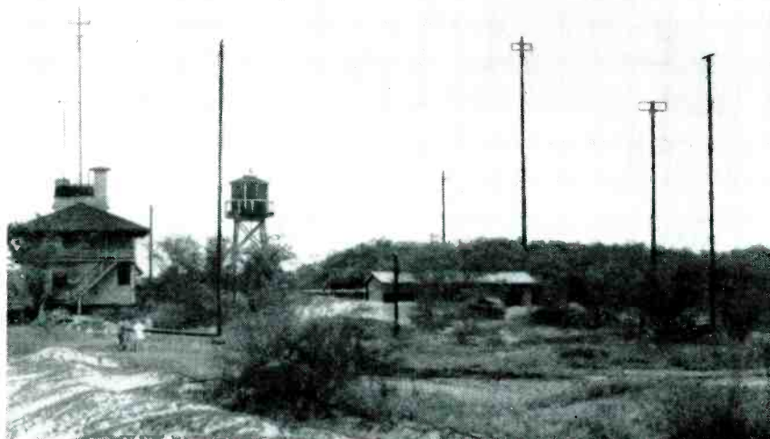
Looking north on the island of Maui, toward Bureau of Standards radio field station. Building at left houses WWVH frequency controls and transmitting equipment. Field crew is completing erection of vertical half-wave 10-mc antenna. Transmitting and recording apparatus for ionospheric propagation measurements occupies low building at right. At extreme right is vertical quarter-wave 5-mc antenna
