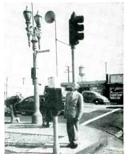
Siren-controlled traffic ear installed in Lynwood, California, has been in constant use since its installation several months ago
