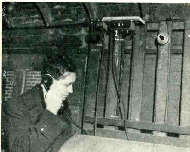
Interior of line car, showing operating position. Busy and call visual signals above and to right of conductor
