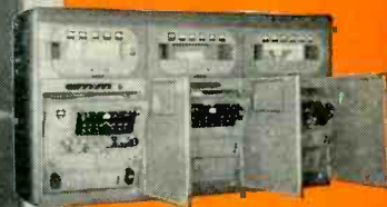
Collins 734A 10 kw FM transmitter installation. Courtesy KKLA, Los Angeles, Calif.
