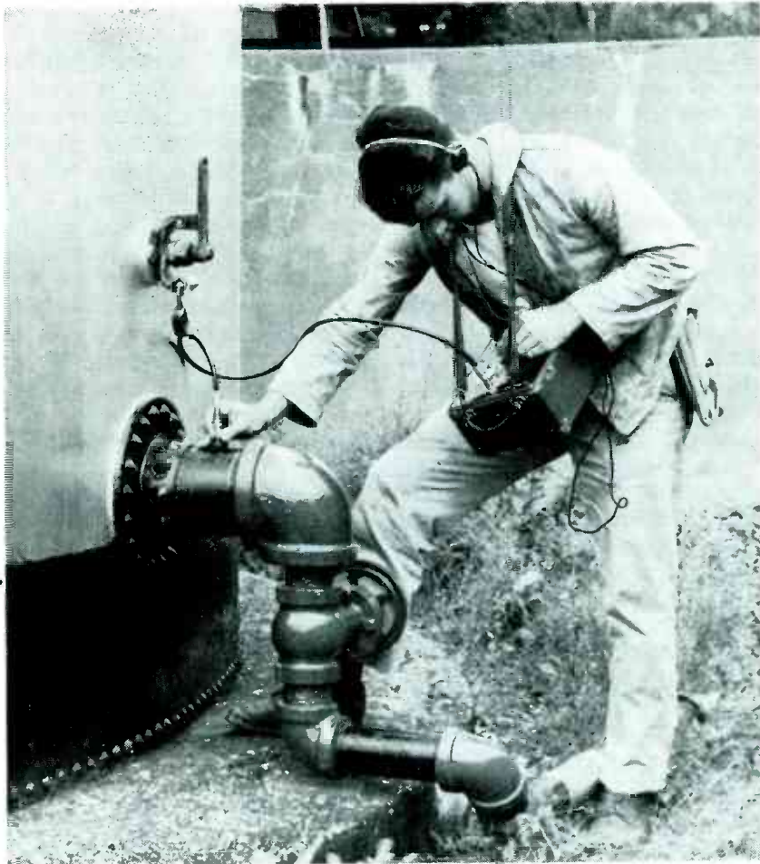
Thickness gage being used to check condition of filled gasoline tank and outlet pipe
