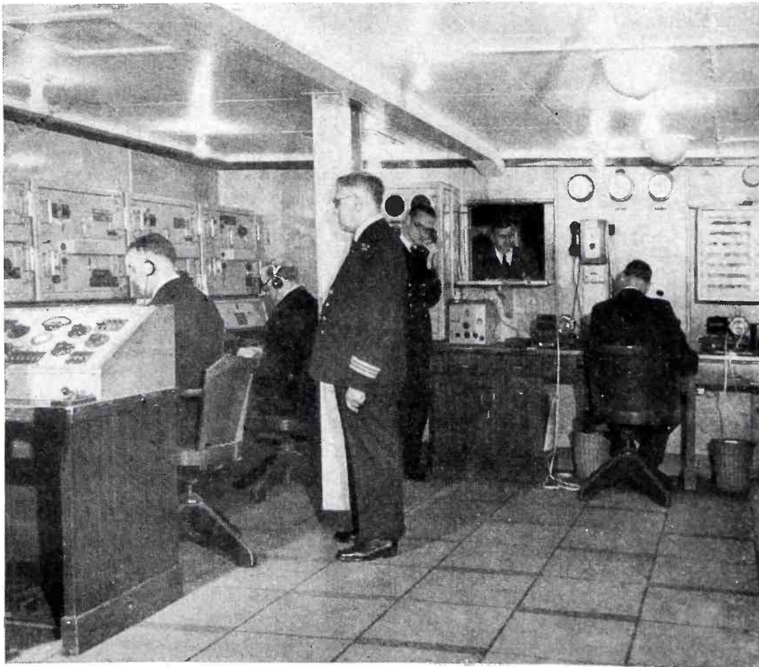
Main radio control room of Queen Elizabeth, showing operating positions and master control desk. The entire marine radio installation was made by International Marine Radio Co. Limited, an I. T. & T. affiliate. Speech secrecy racks fill another wall
