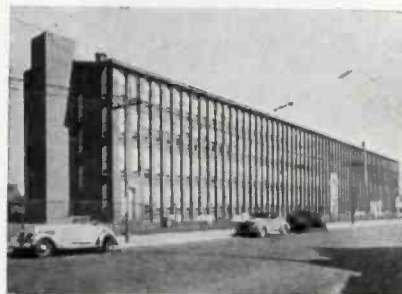
New DuMont plant at Clifton, New Jersey
