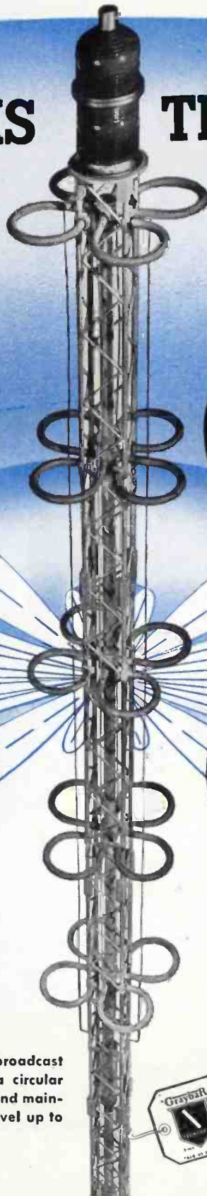
1930 Half-wave vertical radiator, now in general use, was developed into practical form. It greatly improved signal output of broadcast stations.
