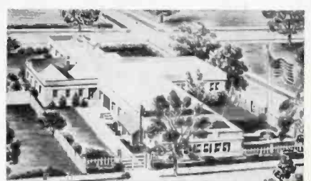
New plant of Essex Electronics
