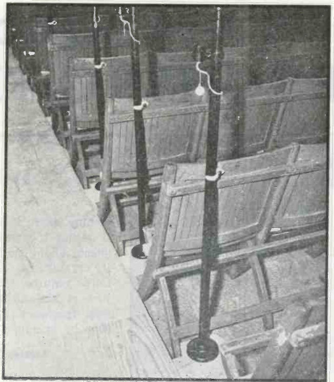
FIG. 3—Method of anchoring delegation microphone stands to backs of seats and to temporary flooring laid in aisles over 3/8-inch wood sleepers
