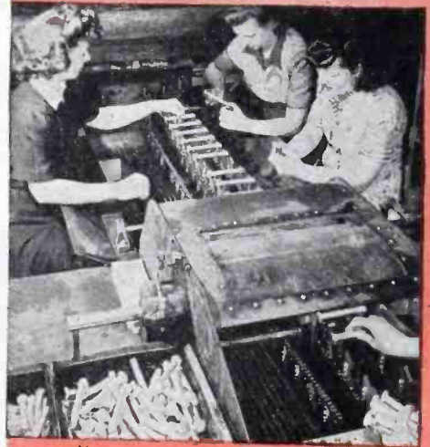
Magnetic inspection by Magnaflux machine.
