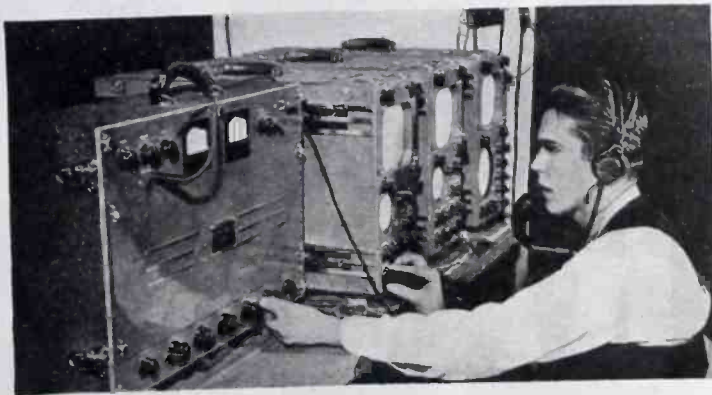
RCA control equipment used by NBC at Madison Square Garden. The audio control unit is at the left, video units at the right, power supply units beneath table. This corresponds to the "remote equipment" used by regular broadcasting stations in outside pickups.
