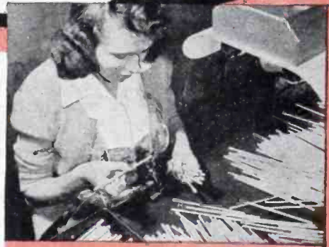
Checking pitch diameters with roller snap gauges.
