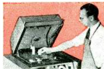
THIS 4-OZ. PIECE of plastic was thoroughly softened for molding in about 15 seconds by an RCA 2000-watt electronic generator.
