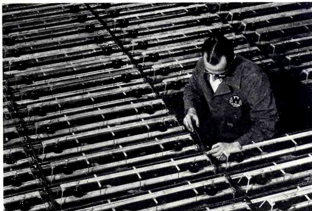
DUST —Electrostatic precipitators designed to rid air of dust and dirt use electronic principles, are more efficient than mechanical filters
