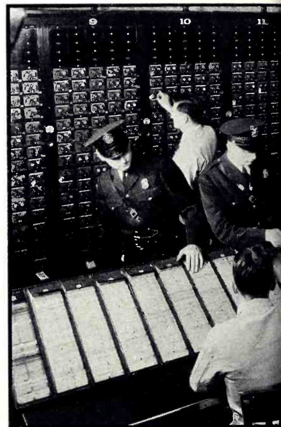
CENTRAL STATION —Men in background watch "drops" remotely operated when trouble occurs on distant protected prem-
