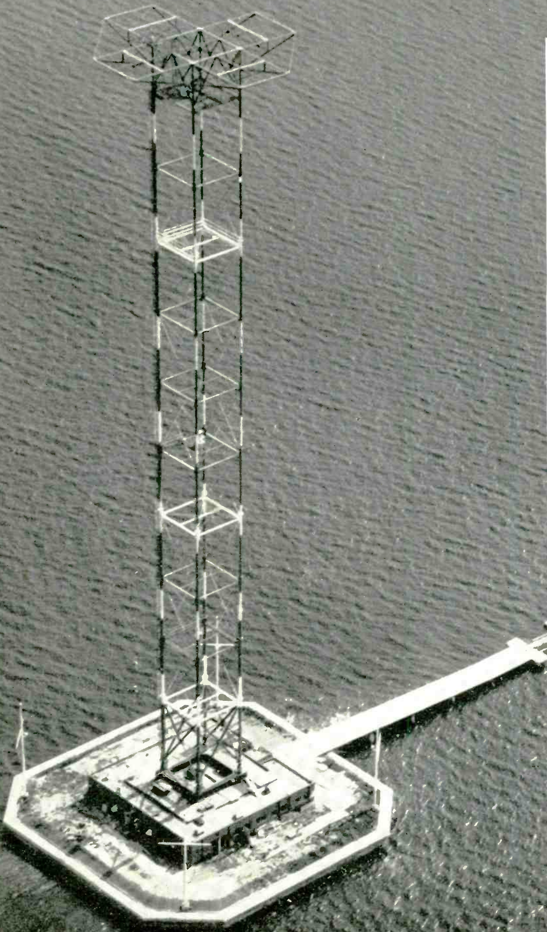
Each corner of the 410-foot antenna structure is supported by a Lapp push-pull tower-footing insulator. Now use of Lapp Fog-type Station Post insulators as stand-off for gas-filled high-frequency lead. Lapp tower footing insulators are available for all pipe masts, self-supporting towers and guyed radiators.
