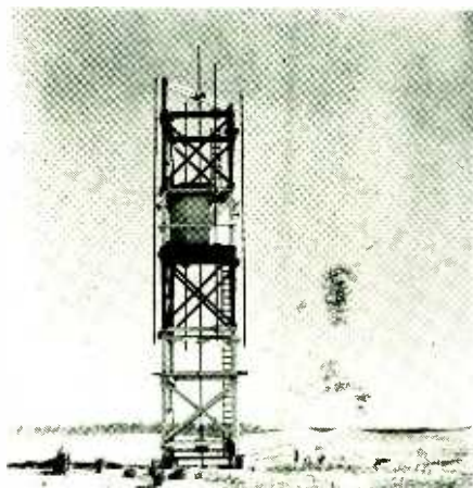
The antenna system is located some distance from the airport and connected to the receiver by telephone lines
