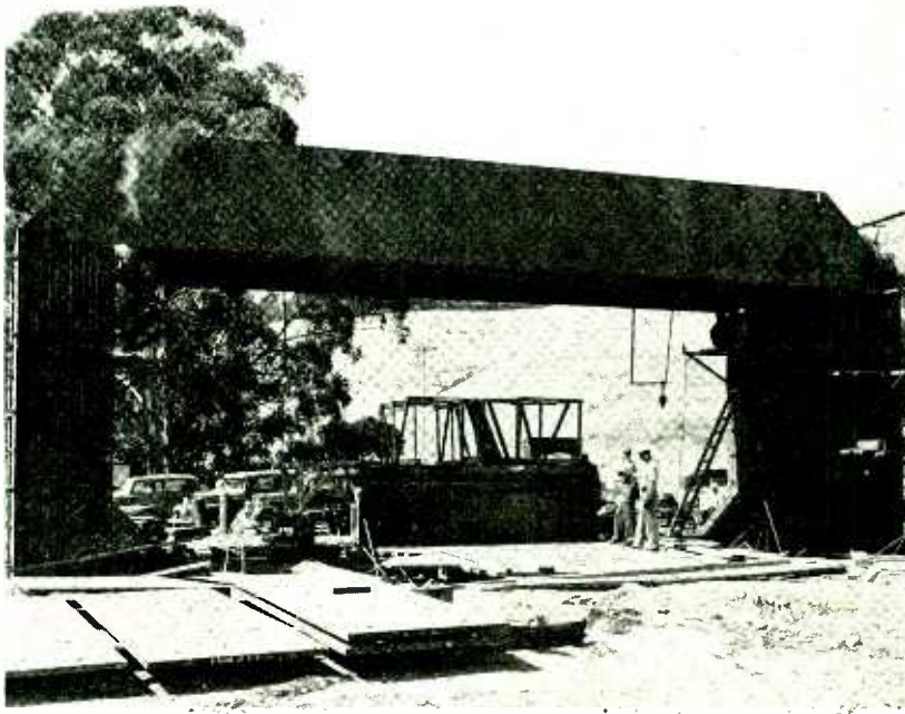
The huge magnet which will be used in the University of California's 4900-ton cyclotron. Some idea of its magnitude can be gained from the relative size of the figures in the foreground
