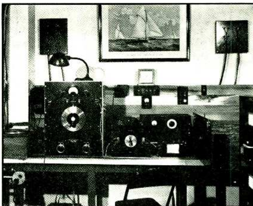
Fig. 4—Audio oscillator and associated equipment used for delivering sound to the subject. The loudspeaker is contained in the sound proof box at the right
