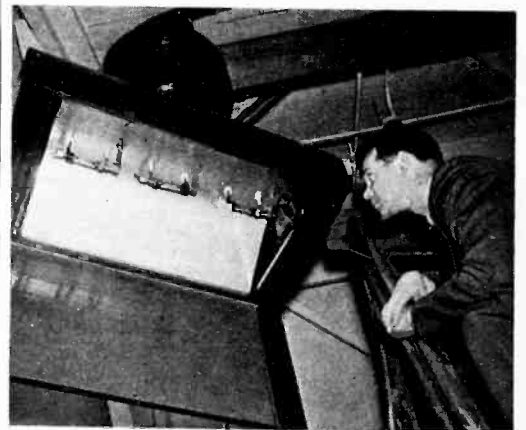
Floodlight unit using three mercury vapor lamps. Because of high intensity and lack of heat, this lighting finds application in black and white television studio work
