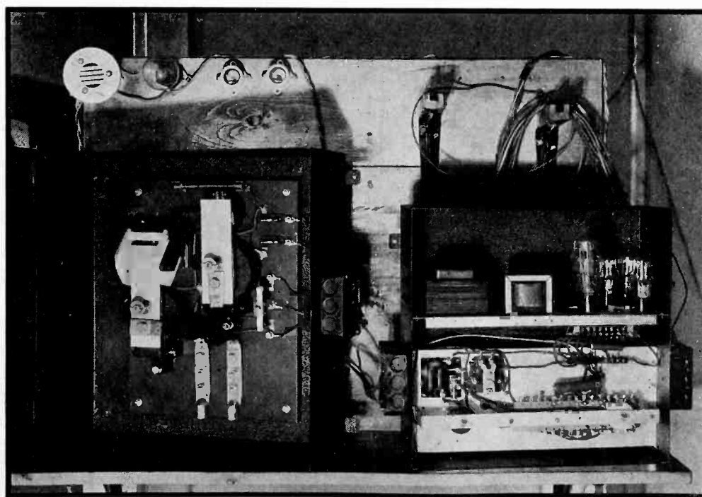
Welding timer "on location"
