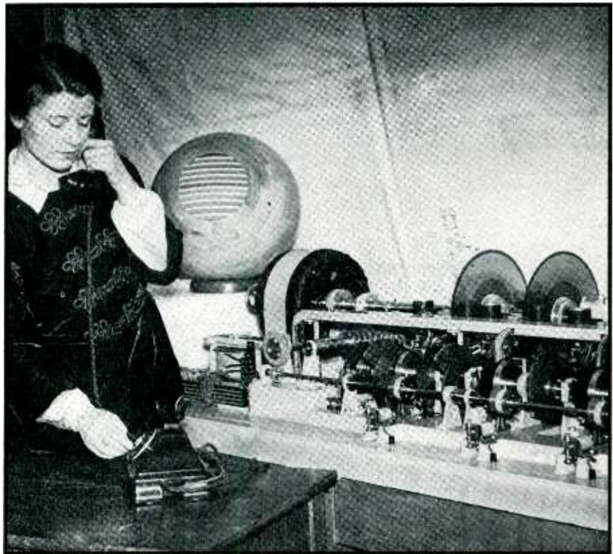
By dialling "T-I-M," British telephone subscribers can connect with this "Talking Clock," which announces the exact time every ten seconds automatically. Circular sound tracks on whirling discs supply the announcement to photocells, which are centered over the required track at the proper instant by a cam mechanism
