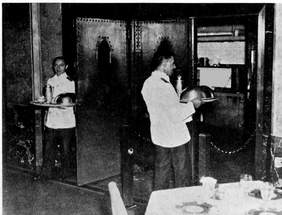
Like many other progressive hotels and restaurants, the Hotel New Yorker, New York City, has installed photo-cell self-opening doors between dining rooms and kitchens. As the waiter walks through a light-beam, the door jumps open
