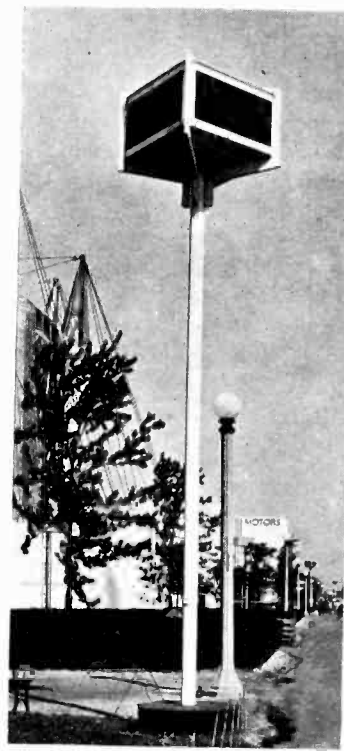
One of the many outdoor loudspeaker sound outlets
