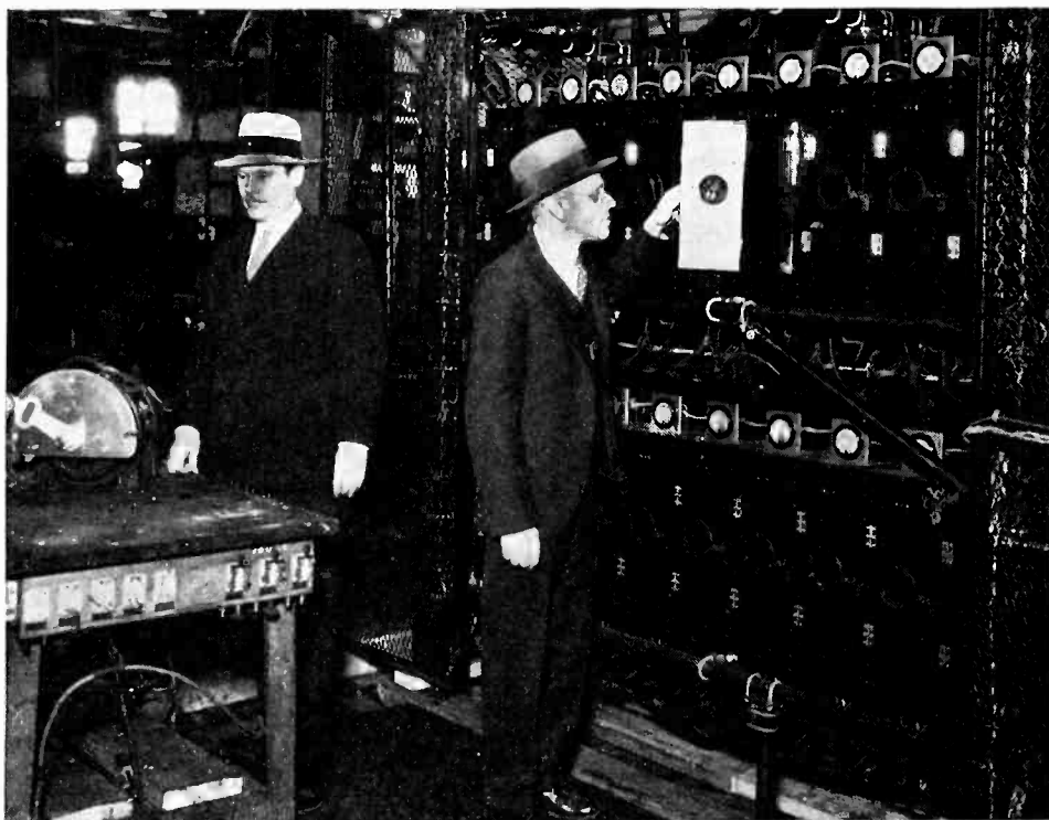
By means of eighteen thyratrons this 400-hp. synchronous motor fed directly from a 4,000-volt line gives ready adjustability in speed
