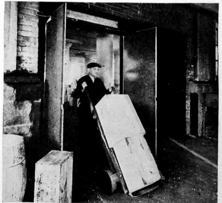
These doors between the shipping room and freight platform of the Stanley Works, New Britain, Conn., are now controlled by a photocell operated by beam of light which shines from floor projector through hole in center of doors (see picture at right). Trucker coming from either direction intercepts beam, silently opening door
