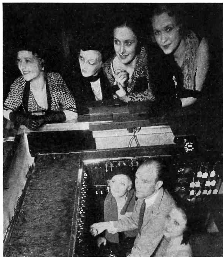
Through thyatron tubes, the fifty lighting circuits in the new Earl Carroll Theater, New York City, are controlled from this keyboard
