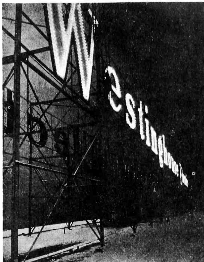
Fig. 8—Large electric sign controlled by photo-electric cells
