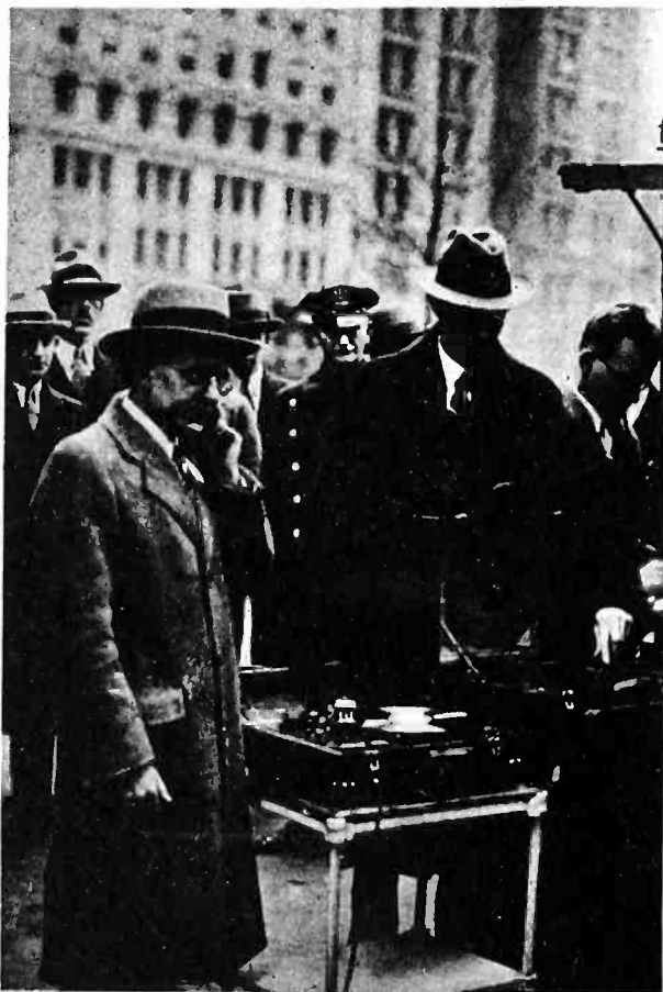
Dr. Harvey Fletcher, sound expert for the Bell Laboratories, measures the noise level in New York City streets
