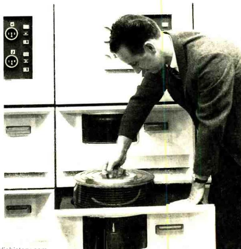
Fig. 3. The disc storage file shown here provides storage for 25 million characters of information.
