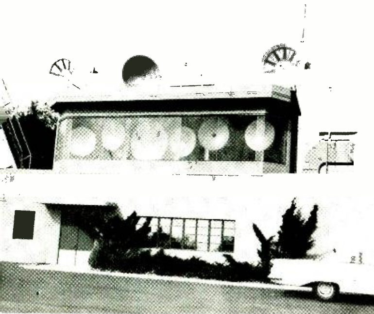
Fig. 3. Weather-shielded microwave antenna housing for studio-to-transmitter microwave relay, photographed at Mt. Wilson, Calif.
