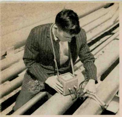
Fig. 7. Portable gamma-ray thickness gage checks pipe walls.
