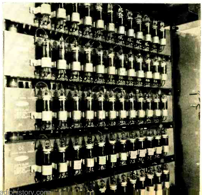
Thyratron tube dimmer bank with 60 tubes providing 30 control circuits. Each dimmer or pair of tubes has a capacity of 5000 watts. The bank shown is approximately 80" wide and 80" high.
