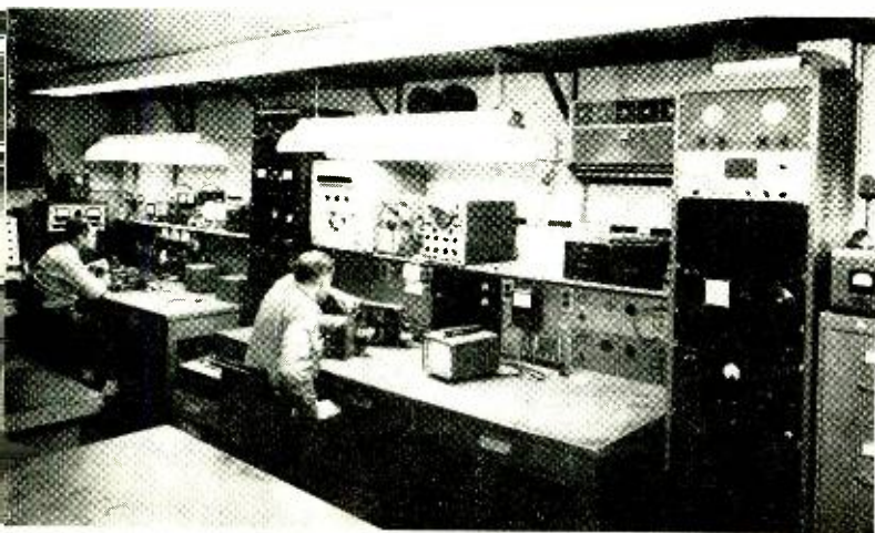
Fig. 7. This is just one corner of the electronic maintenance shop. A closed-circuit TV camera is being repaired. Equipment includes scopes, modulation monitors, deviation meters, frequency meters, wattmeters, and a WWV receiver.
