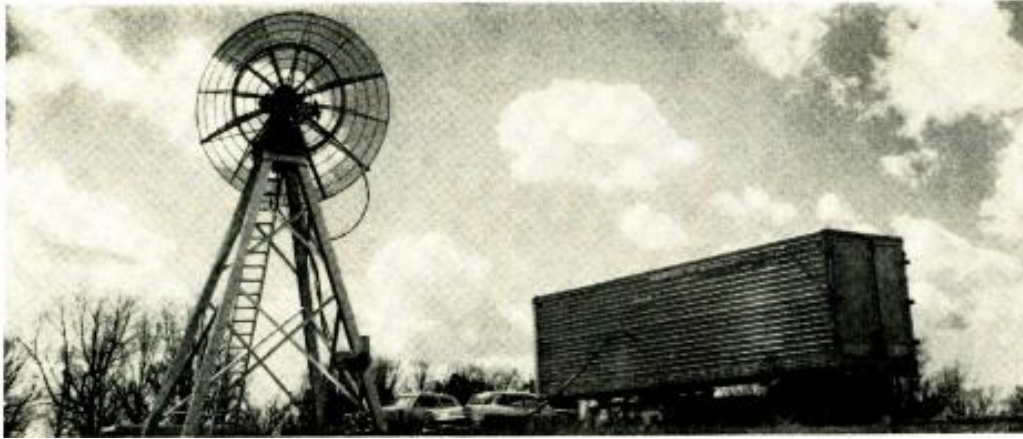
A 14-foot parabolic dish antenna scans the sky while inside the trailer-housed station Army Ballistic Missile Agency engineers receive "Pioneer IV's" signals.
