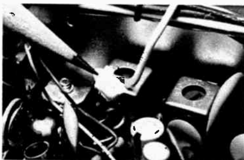
Fig. 2—Signal from adaptor is capacitively coupled into IF strip by cementing wire from adaptor to IF can with GE silicone adhesive.
