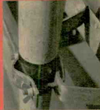
Fig. 12—Standard wall bracket supports mast 2-ft. above base. Insulate mast with electrical tape.
