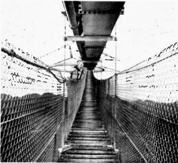
A catwalk goes from base of a support tower to feed-support structure. Rectangular object at top of the photo is the signal-carrying waveguide.
