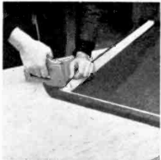
Grille cloth, open-weave burlap, is being stapled to wood frames.
