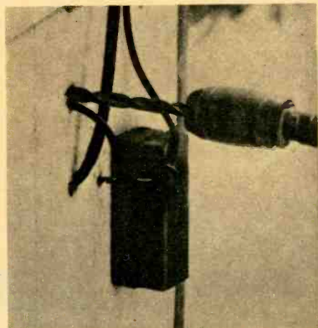
Fig. 1—Drill hole for the coax at an upward angle from the outside. Wire through standoff is short-wave antenna lead-in and has loop to prevent water from entering house. Other wire is for phone.
