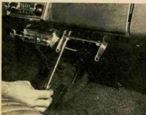
Only two No. 8 self-tapping screws were required to install bracket for typical solid-state transceiver. You start holes with punch, then drill.
